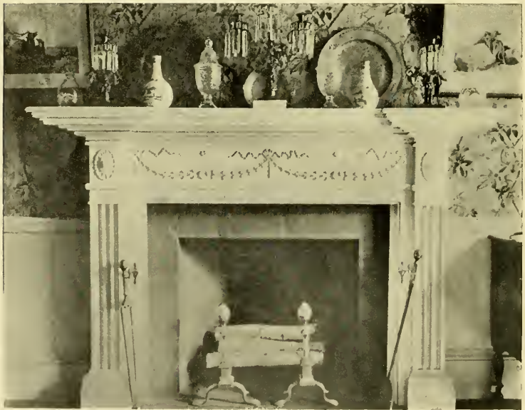
PLATE LXXVII. — Soapstone Fire Frame, Kittredge House - Fireplace, Kittredge House.
